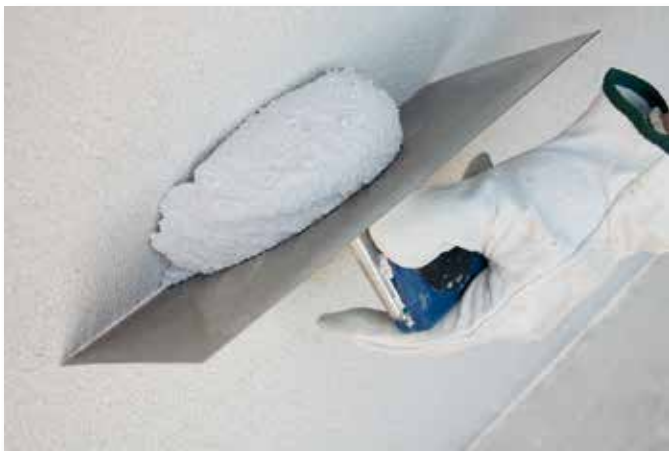
Application using a smooth-edged trowel
