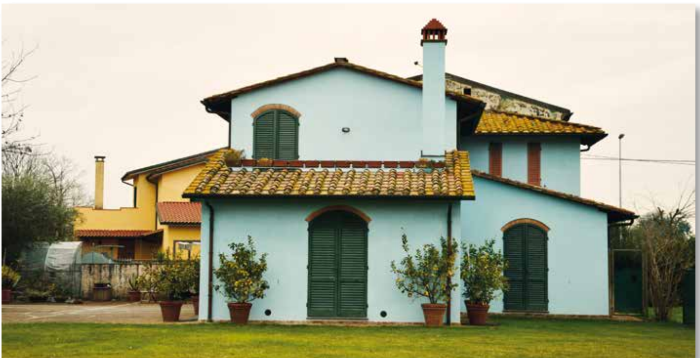
PISA: Facade treated with AFONTERMO®
