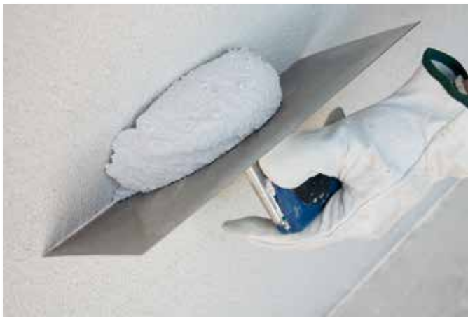
Application using a smooth-edged trowel
