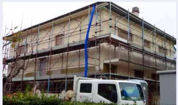
External facade of a building at Navacchio (PI)
